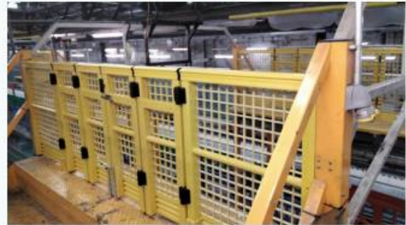
Measured grating extension fitted into the existing gantry arrangement.
