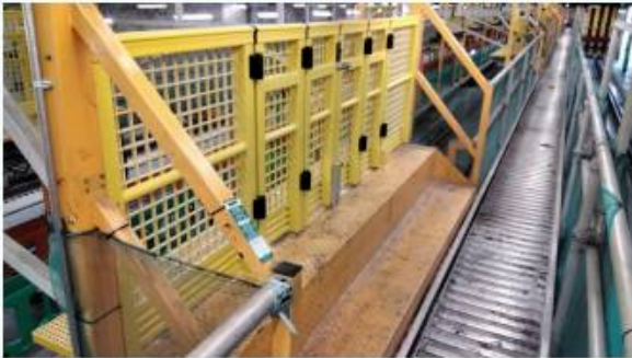
The extension detail was fitted to retained framework and grating rather than treated as a standard new-build platform.
