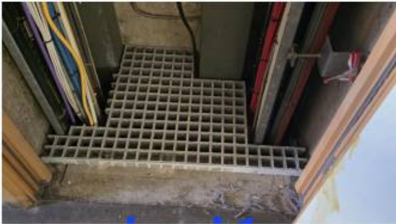
A typical tower-level infill showing the GRP panel, surrounding riser services and local fixing condition.
