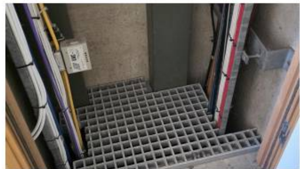
Level 6 installation showing the repeated support and fixing approach.
