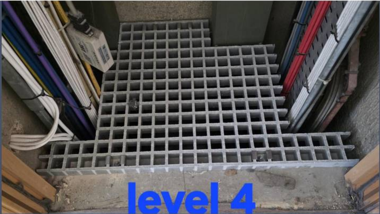
Level 4 Infill coordinated around the riser opening.
